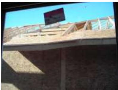
Oh oh, the roof trusses don't seem to line up here – the cause, the garage and home walls were not framed to the same height!
