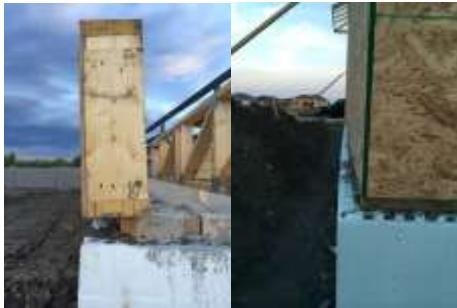
In these pictures, one wall is barely sitting on the foundation of the home and the other is incredibly crooked. Accurate foundations and framing are vital to the build.
