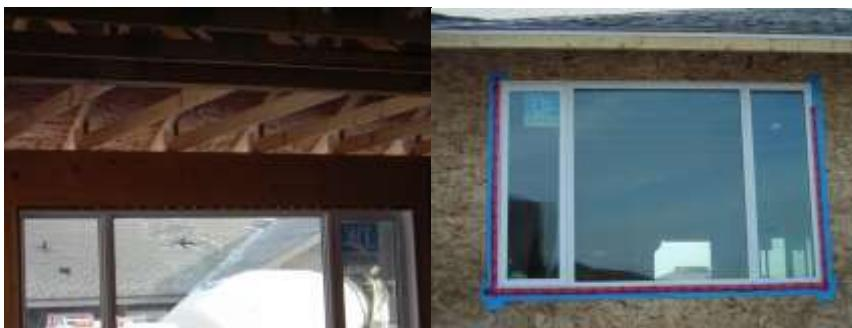
This shows a window that has not been properly installed – there is nothing securing the top of the window to the wall and the builder is clearly done as they have blue skinned and tuck taped the exterior of the window.
